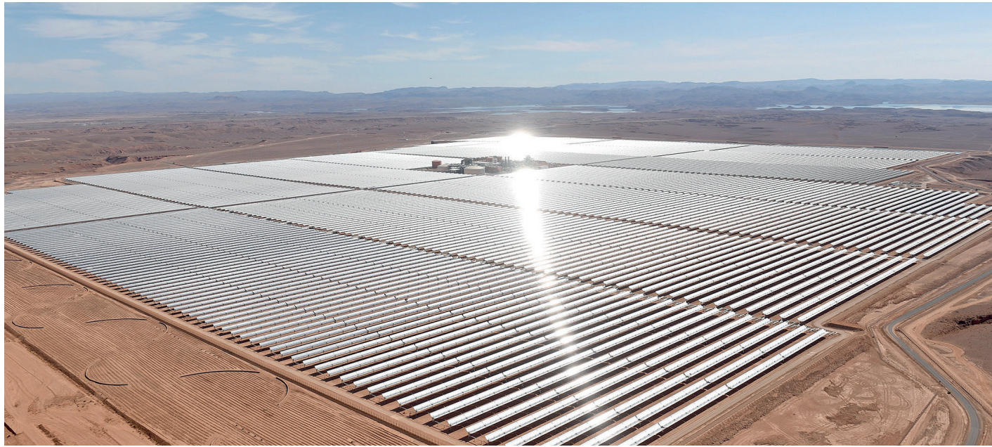
Morocco has accumulated a total renewable energy capacity of around 4.6 gigawatts. This includes 1,853 megawatts in wind power, with an investment of almost 30 billion Dirhams, and 852 megawatts in solar power, with an investment of around 30 billion Dirhams
