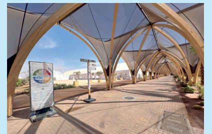
Al Haouz construction sites Land marked out
