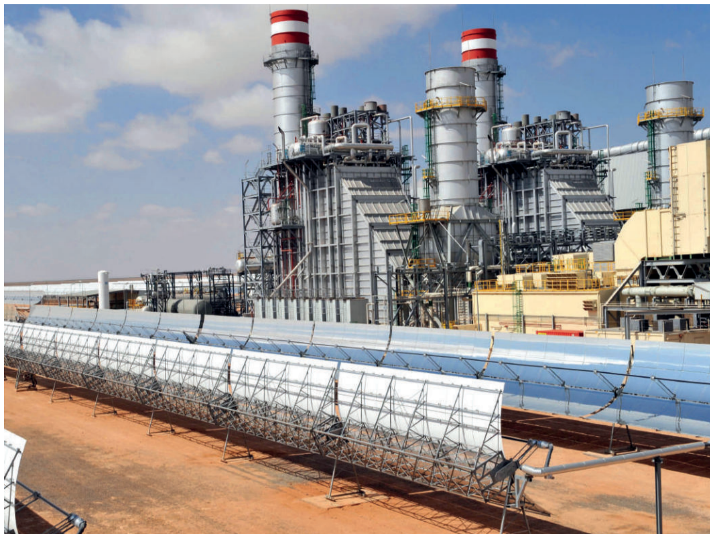
Morocco's national energy efficiency program targets the building, industry, transport, agriculture, and public lighting sectors, which together account for 90% of the country's energy consumption. Through 80 concrete measures, the program aims to achieve energy savings estimated at around 20% by 2030 (Ph. D.R.)
